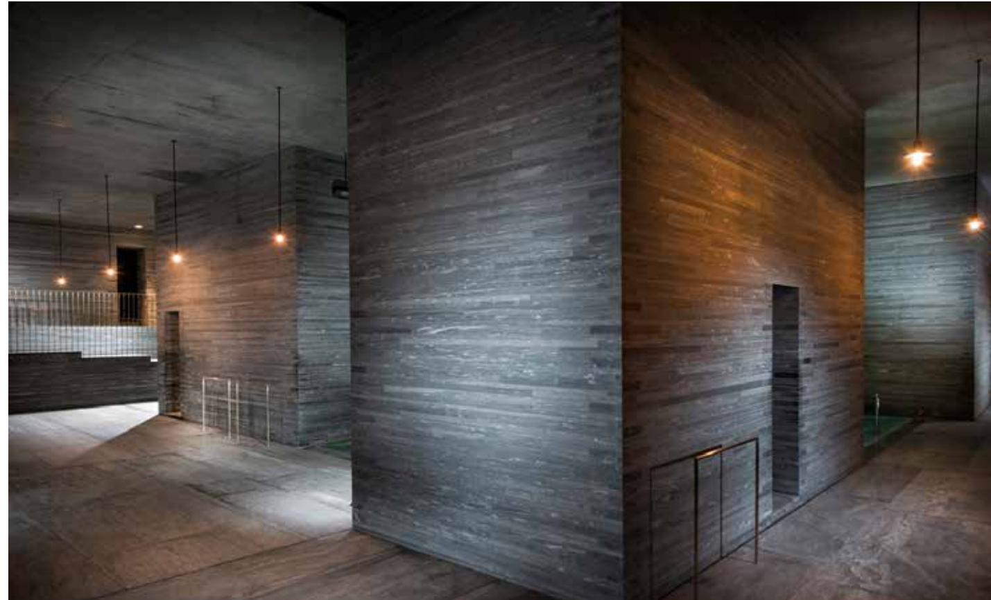
ENTRANCES TO THE INDOOR BATH. THIS IMAGE ALSO SHOWS THE LOCALLY QUARRIED VALSER QUARZITE SLABS THAT ARE LAYERED UP ON ALL THE WALLS.
