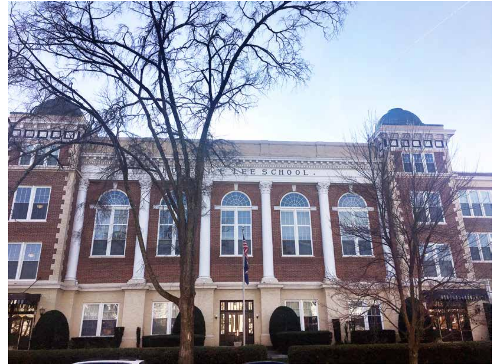
3101 KENSINGTON AVE | FRONT VIEW FROM KENSINGTON AVE
