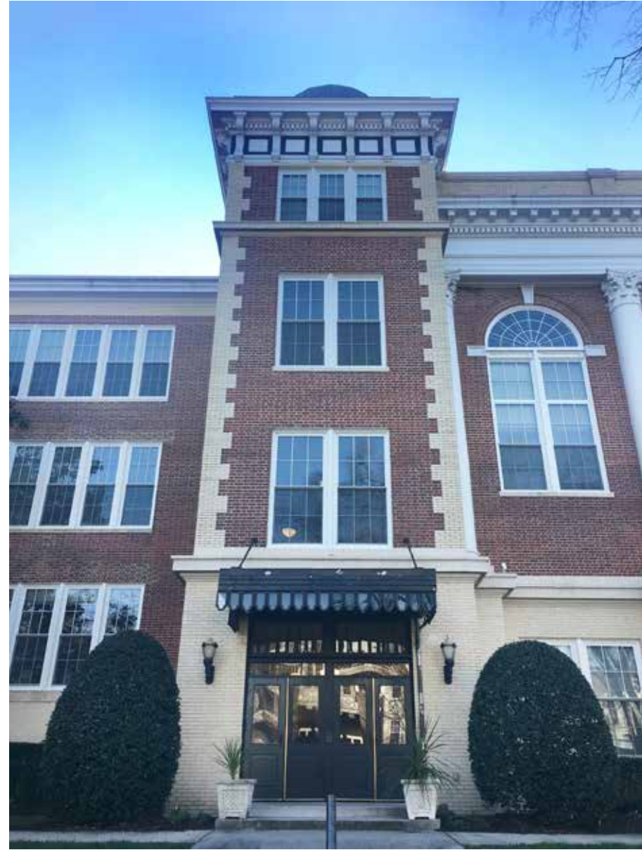
ONE OF TWO FRONT TOWERS
